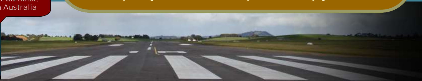
Working on the Mount Gambier Airport runway resurfacing project
